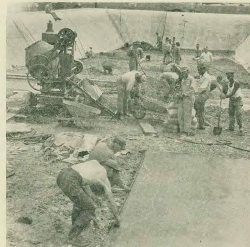
Enlisted men of Strother Field are shown above working in the swimming pool, completing the laying of the concrete floor. The EM are responsible for 90% of the labor on the pool, according to Capt. Oren P. Stoner, athletic director.
