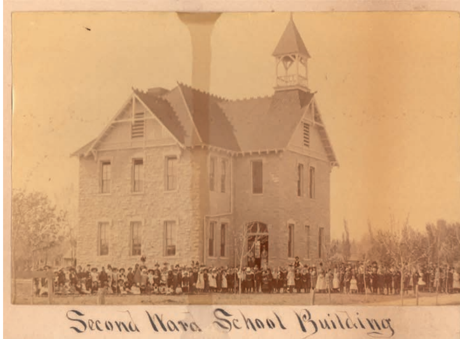
The oldest known photo we have of our building, the Second Ward School, taken by early Winfield photographer Hezekiah Beck.
